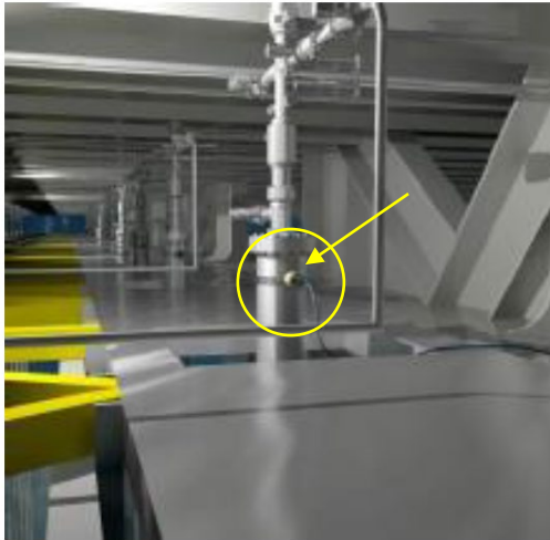
Figure 21—Illustration of sensors mounted on conductor of the well
